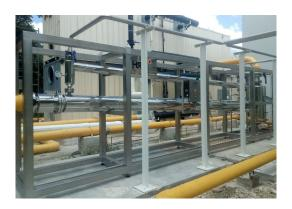
The HRS BDS Series is an efficient solution to cool and dehumidify biogas for combustion with two standard options. The system condenses up to 90% of the water contained in the gas, which is continuously separated before the lean biogas is ready for use. This is a necessary process for all bio-energy plants that use biogas as fuel in CHP engines.
